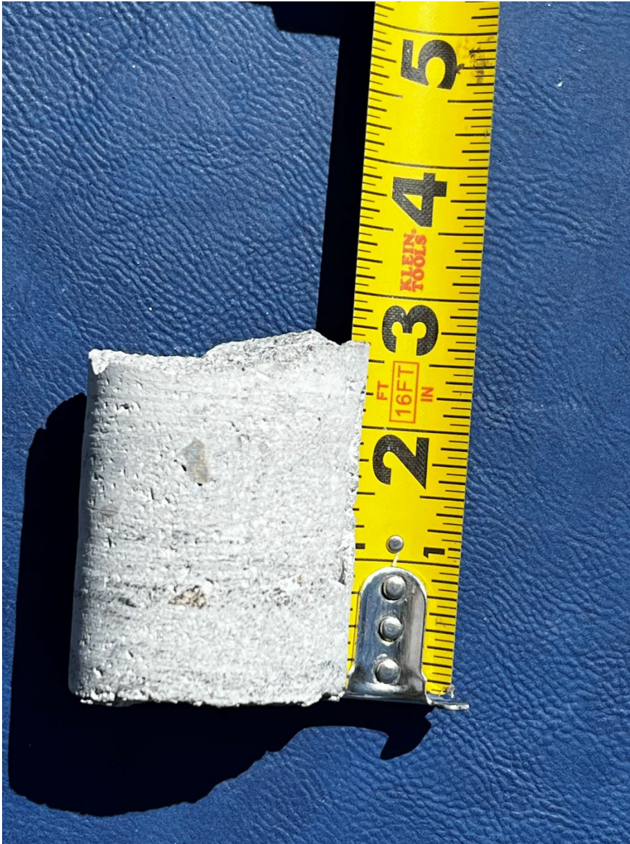
Recovered core was 2.75-inches long and appeared to be sound and competent. No damage to concrete observed.
