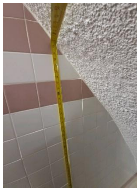
FIGURE 79: HEADROOM CLEARANCE HEIGHT
