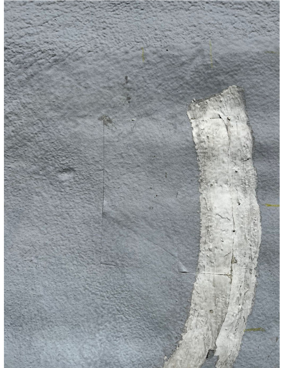
Core location after patching.
