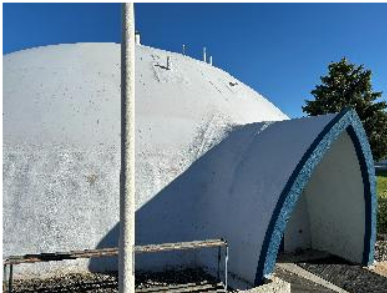
FIGURE 42: TYPICAL COVERED ENTRANCE AT SMALLER DOMES.
