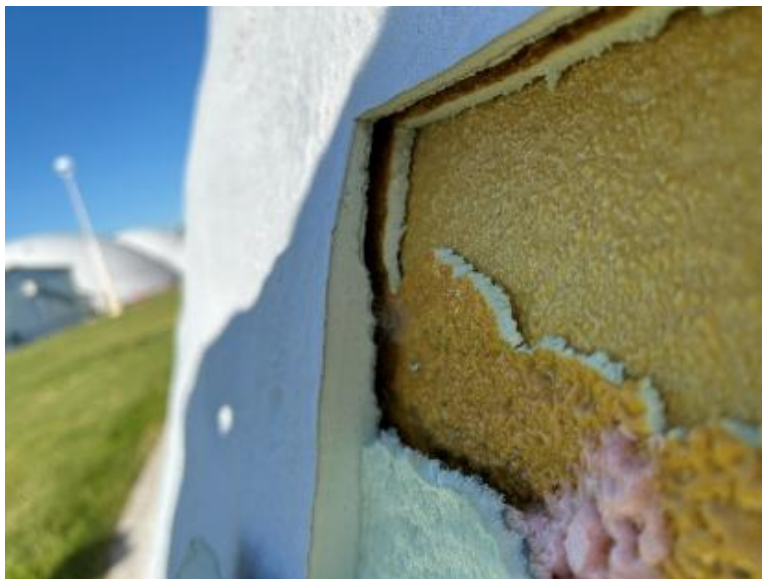
FIGURE 31: LAYERS OF FOAM INSULATION AT EXPLORATORY OPENING.
