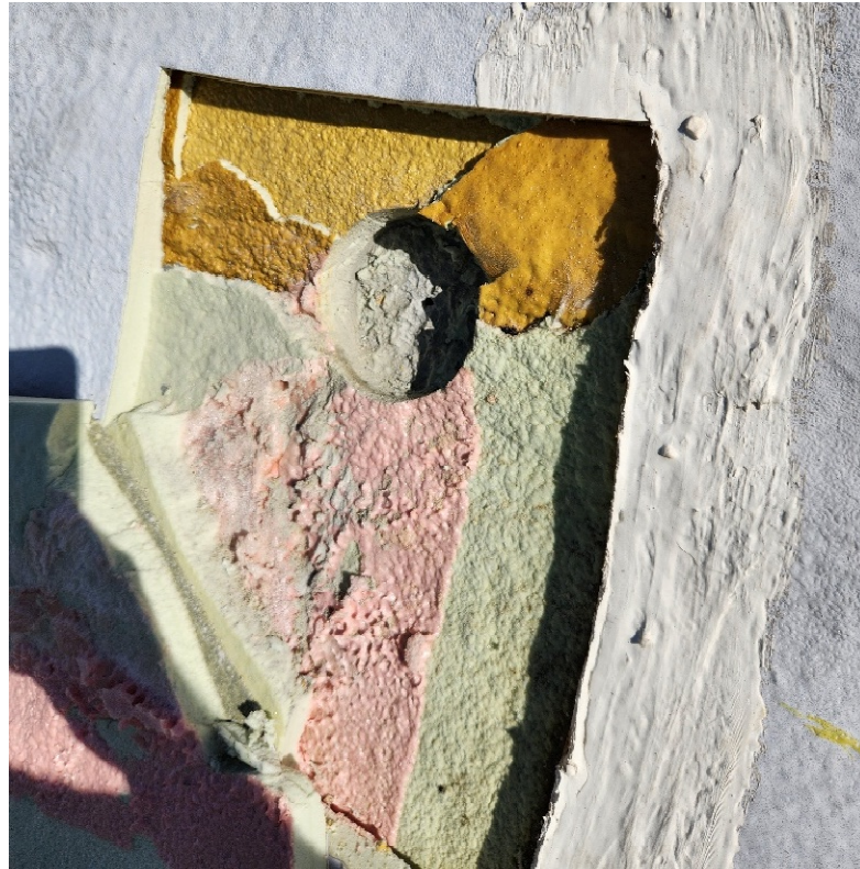
FIGURE 27: DOME A EXPOSED ENVELOPE
