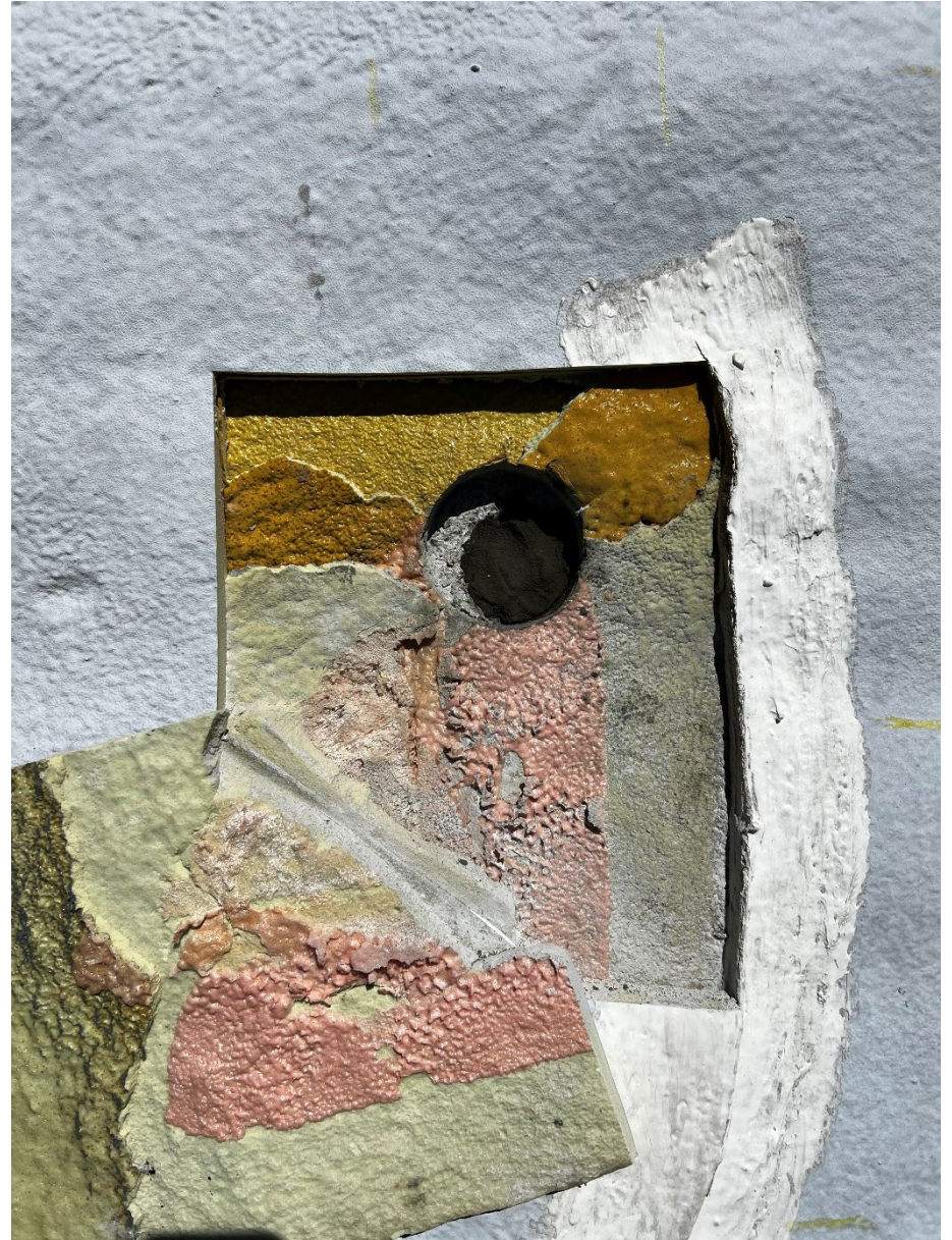
Hole was patched with fast-setting packaged non-shrink grout.
