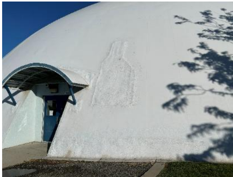
FIGURE 6: REPAIRED ROOF AREA ON DOME #1.
