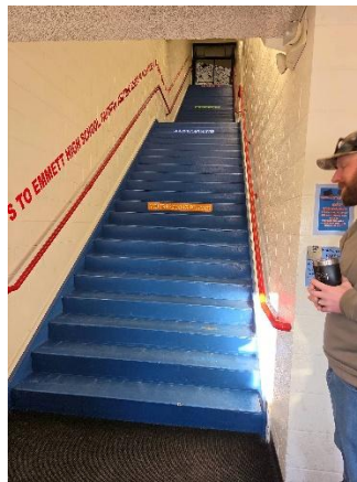
FIGURE 70: STAIRS LOCATED IN MAIN ENTRY VESTIBULE
