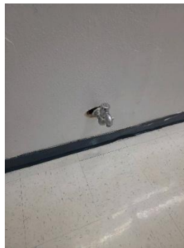
FIGURE 52: MISSING ESCUTCHEONS
