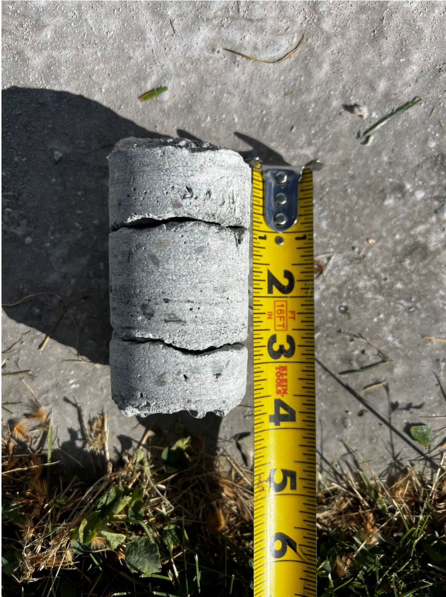
Recovered core was 3.5-inches long and appeared to be sound and competent. No damage to concrete observed.
