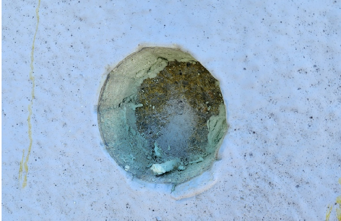
FIGURE 29: DOME B EXPOSED ENVELOPE
