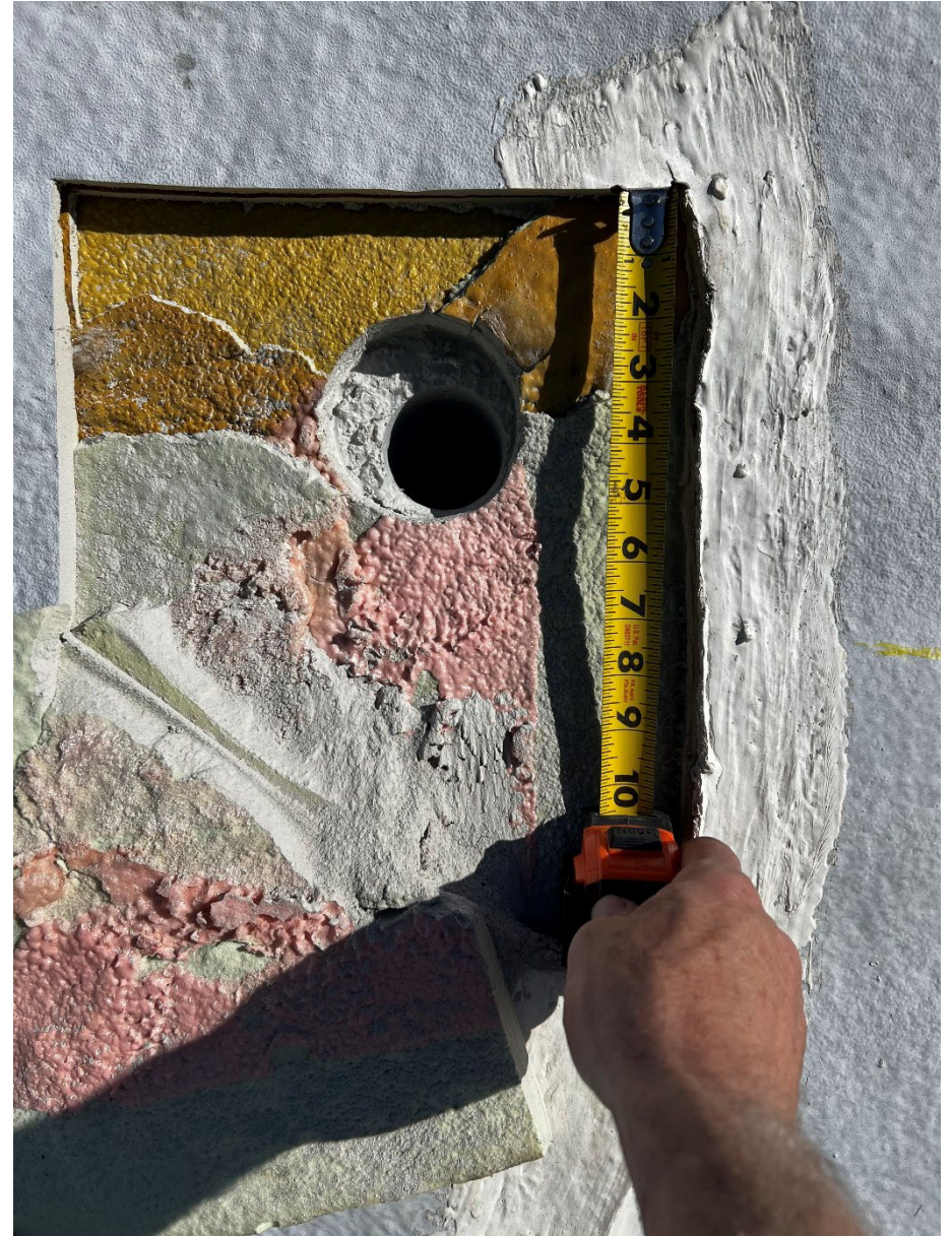
Core advanced through foam and then through concrete.
