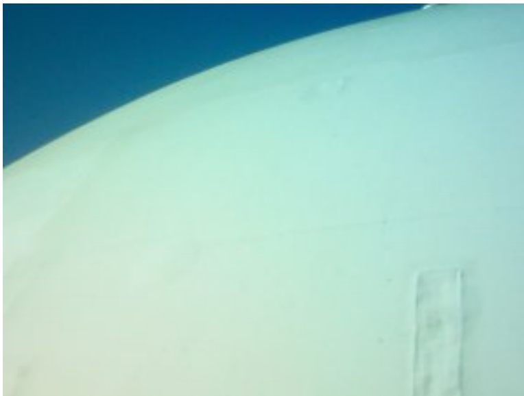
FIGURE 10: AREA OF DOME #1 WITH PATCHED AREA OF ORIGINAL ROOF MEMBRANE.
