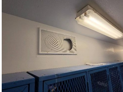
FIGURE 45: REMOVED SPEAKERS
