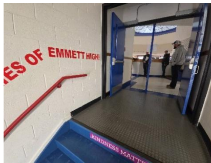
FIGURE 94: STAIR HANDRAIL EXTENSION
