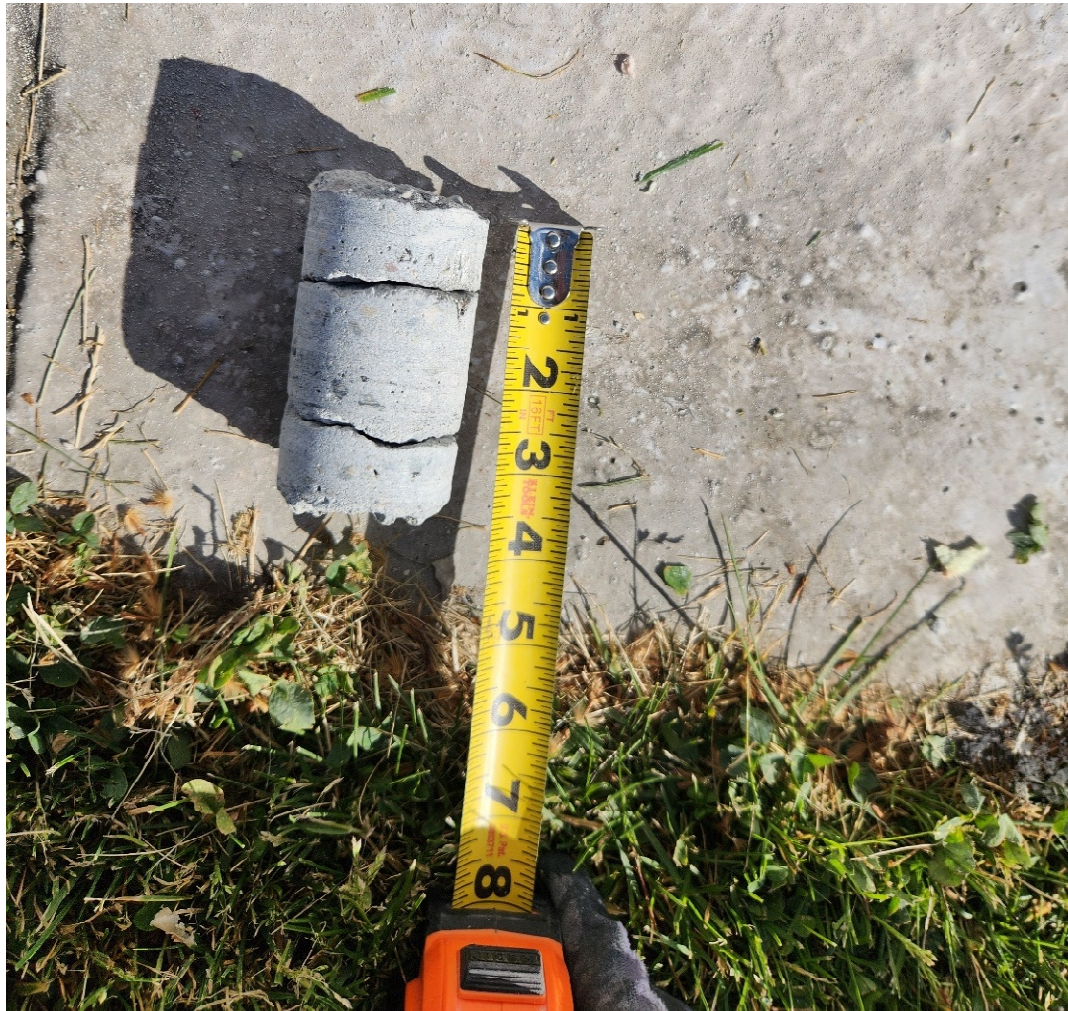
FIGURE 26: DOME A CONCRETE SAMPLE
