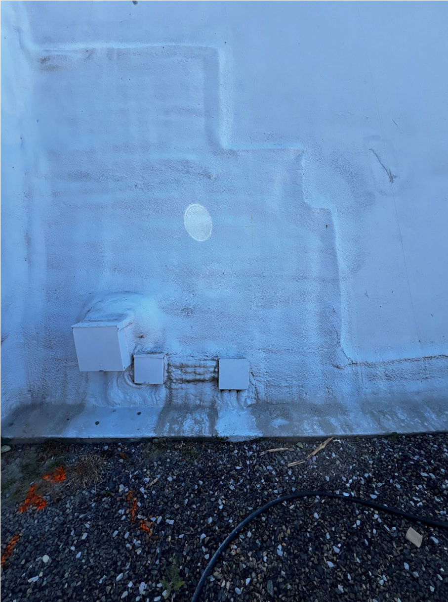
Location of core sample at Dome A.
