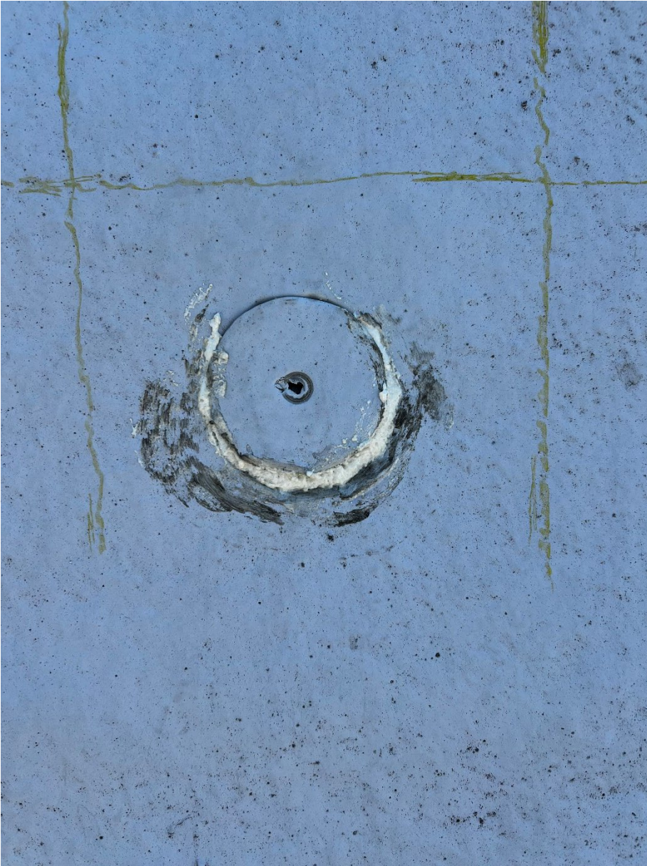
Membrane was re-adhered using spray urethane foam.
