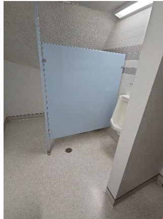
FIGURE 85: MEN'S STAFF RESTROOM
