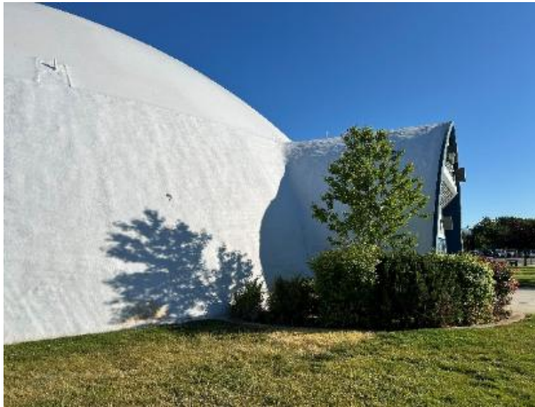
FIGURE 2: REPAIRED ROOF SYSTEM AT BASE OF DOME #2.
