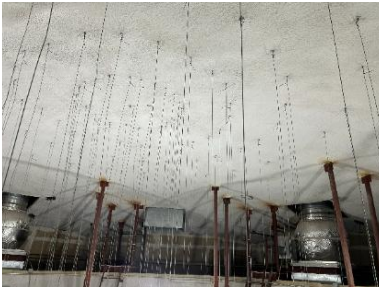
FIGURE 36: UNDERSIDE OF TOP OF DOME #1 IN SERVICE AREA ABOVE FAUX ATRIUM.
