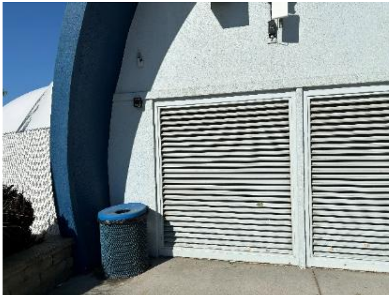
FIGURE 49: TYPICAL LOUVER ASSEMBLY INSTALLED IN VERTICAL WALL.
