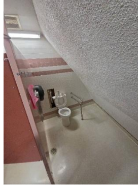
FIGURE 78: HEADROOM CLEARANCE AT STAFF RESTROOM
