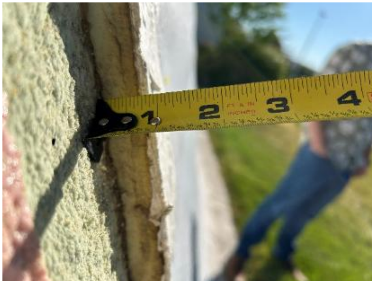
FIGURE 33: FOAM INSULATION ADDED DURING 2012 REPAIR.
