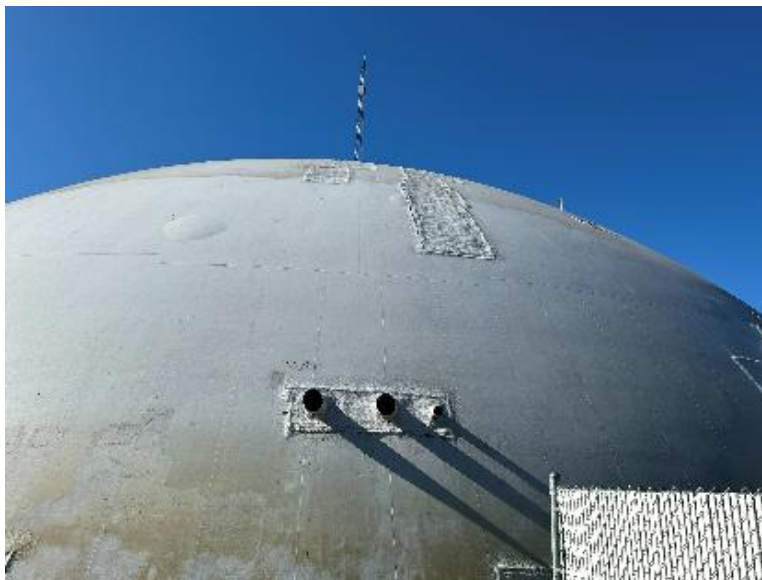
FIGURE 3: ROOF REPAIRS AT PENETRATIONS AND THE UPPER PORTION OF DOME #1.
