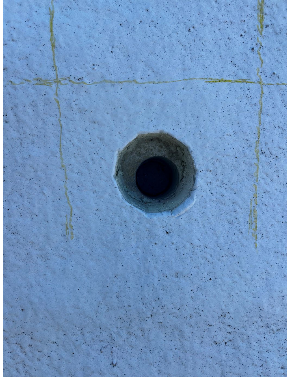
Roof membrane was cut with a hole saw and pried out.
