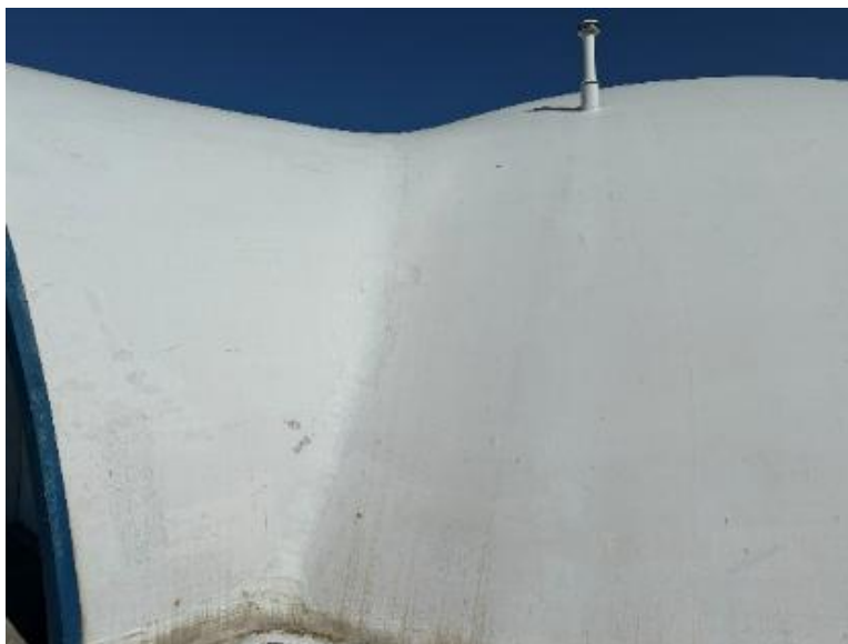
FIGURE 12: AREA OF DOME #5 WITH ORIGINAL ROOF MEMBRANE.
