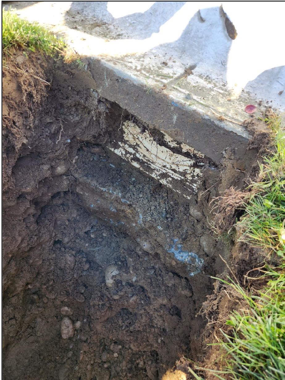
FIGURE 22: DOME “B” FOUNDATIONS AT EAST SIDE OF THE DOME
