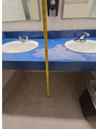
FIGURE 57: WORN BATHROOM COUNTERTOPS
