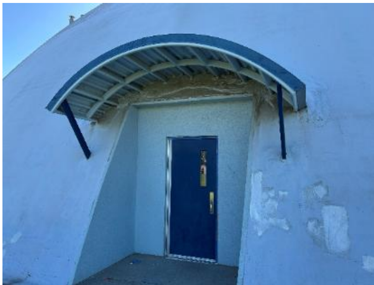
FIGURE 38: TYPICAL SECONDARY ENTRANCE AT ALL DOMES.
