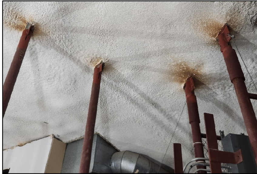
FIGURE 1: CATWALK SUPPORT ATTACHMENT TO PRIMARY DOME STRUCTURE
