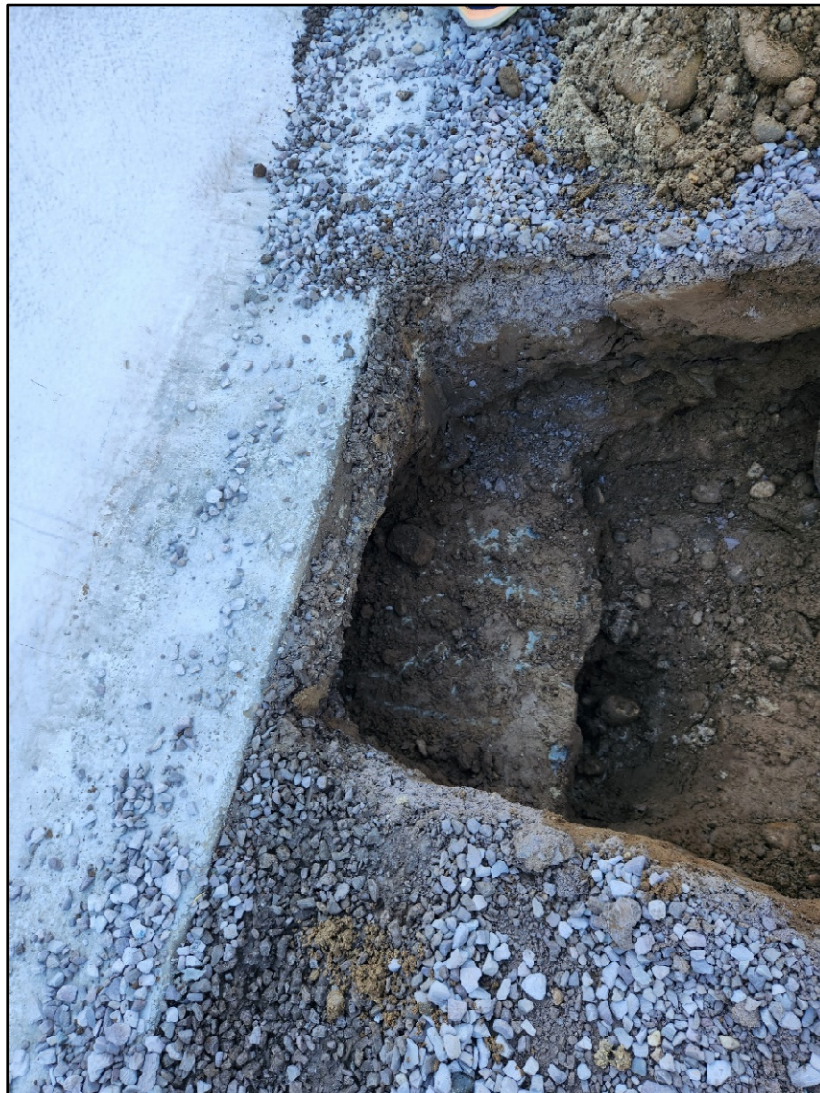
FIGURE 20: DOME “A” FOUNDATIONS AT SOUTHWEST SIDE OF THE DOME
