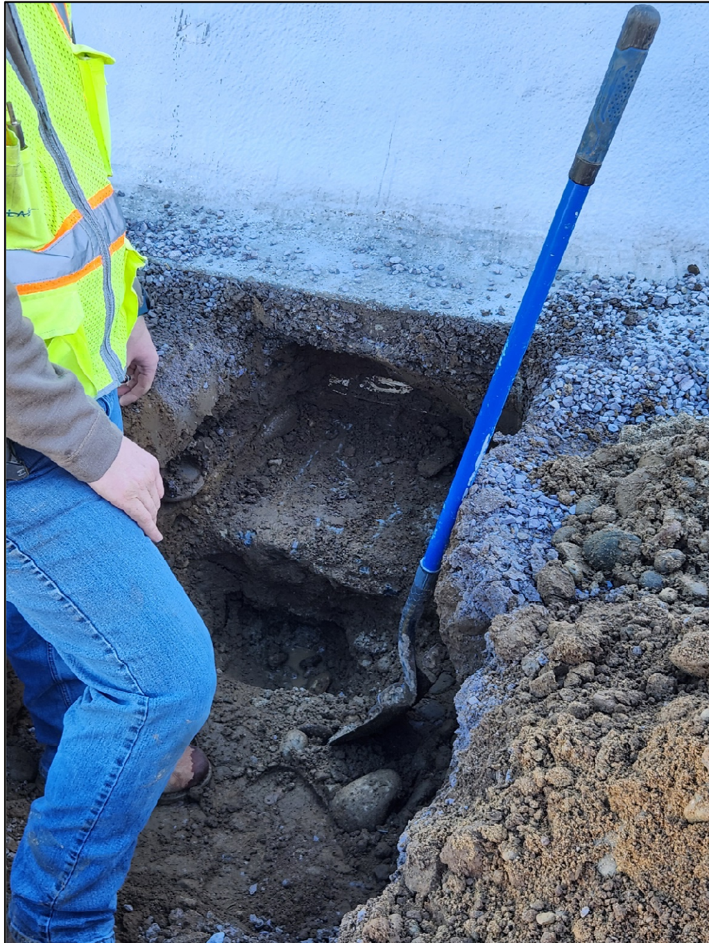
FIGURE 21: DOME “A” FOUNDATIONS AT SOUTHWEST SIDE OF THE DOME
