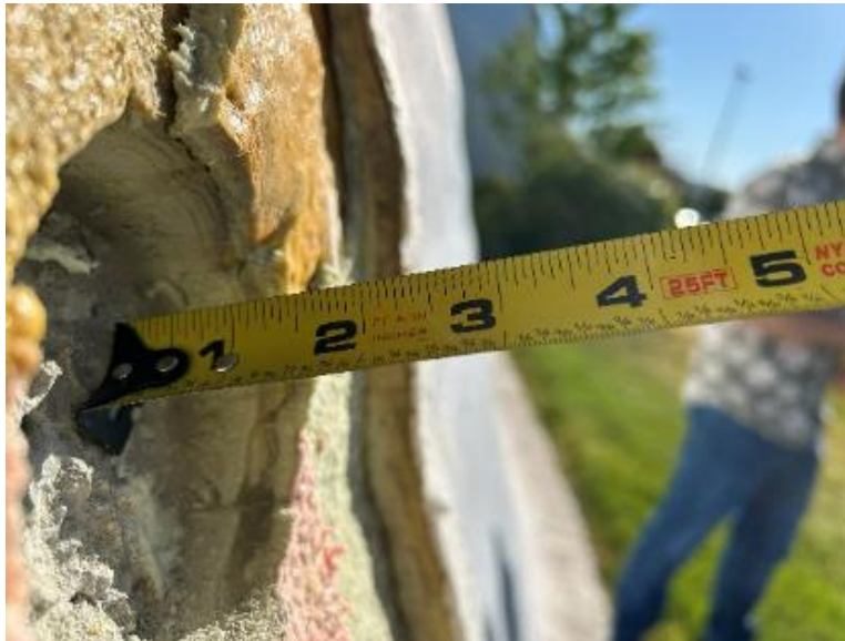
FIGURE 32: DEPTH OF FOAM INSULATION AT EXPLORATORY OPENING.
