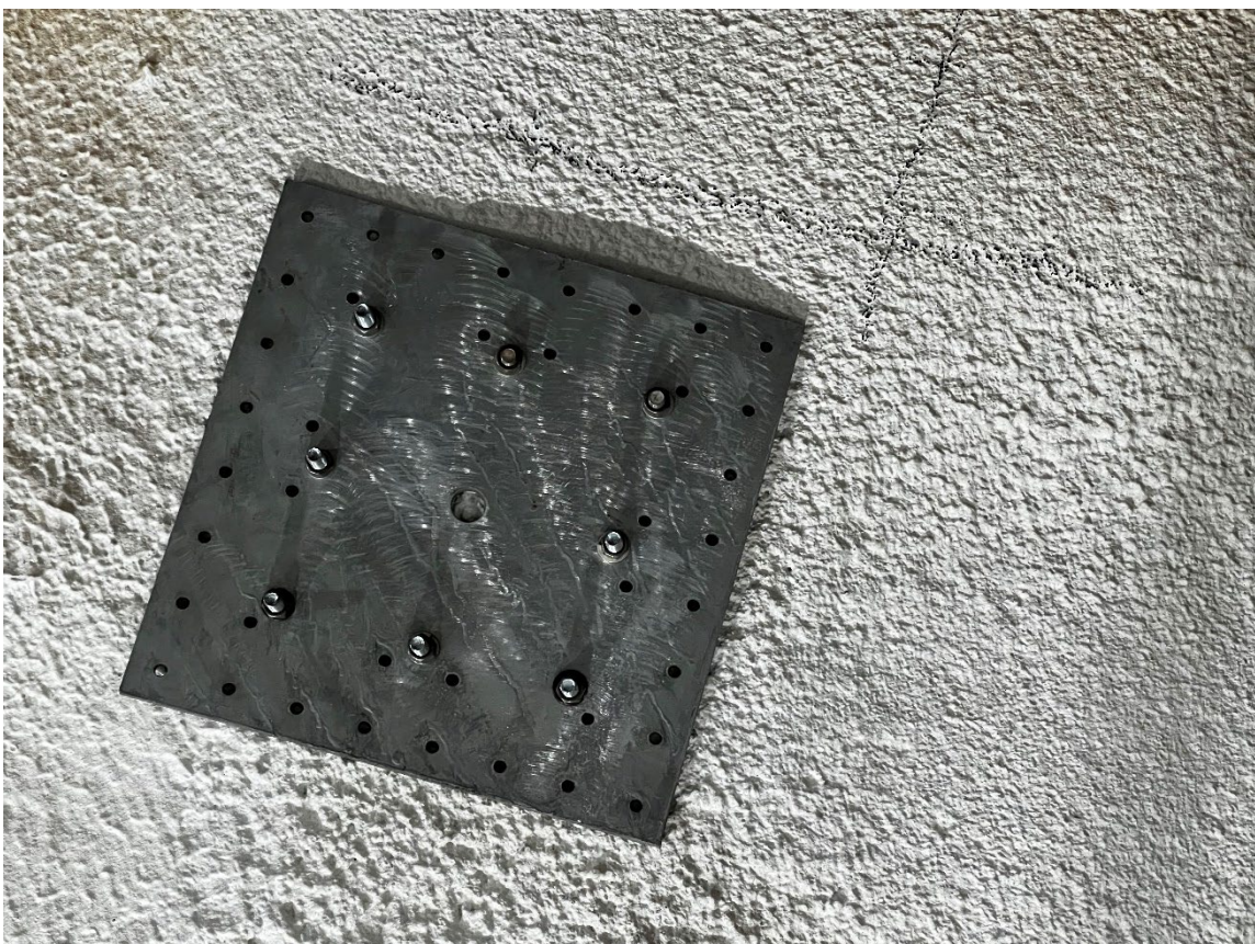
Location 4 clockwise from entry. All concrete sound. No damage. Plate installed for roof anchors.
