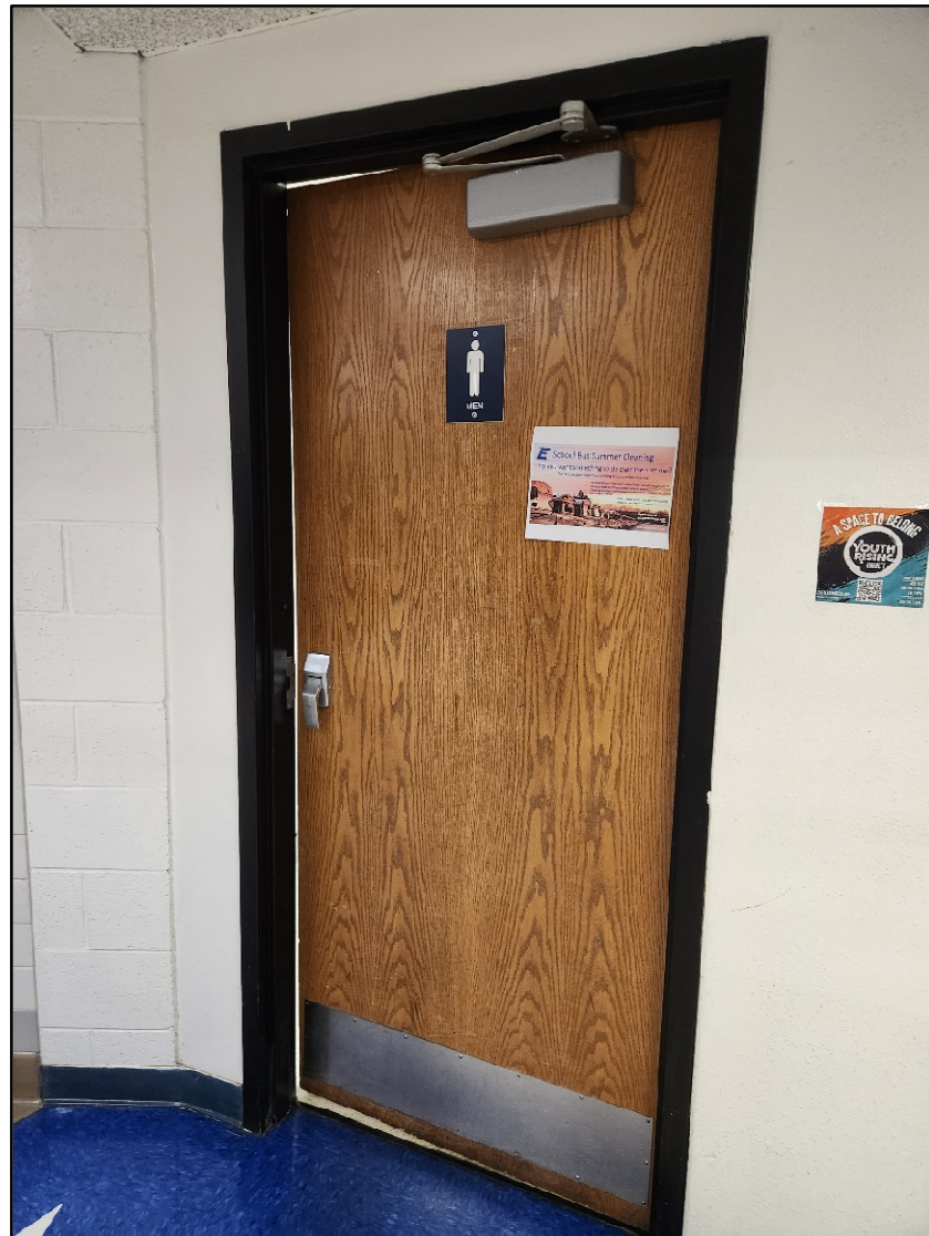
FIGURE 6: MEN'S RESTROOM DOOR AT LEVEL 2
