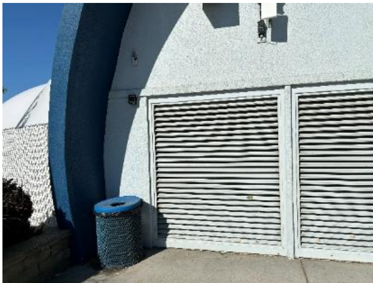
FIGURE 40: TYPICAL LOUVER ASSEMBLY INSTALLED IN VERTICAL WALL.
