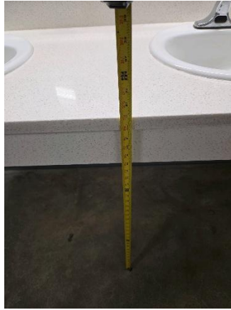
FIGURE 89: RENOVATED BATHROOM COUNTEROPS
