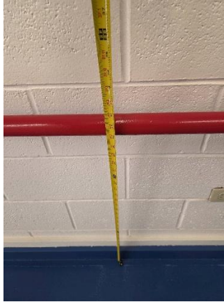
FIGURE 96: HANDRAIL HEIGHT AT MAIN STAIRS
