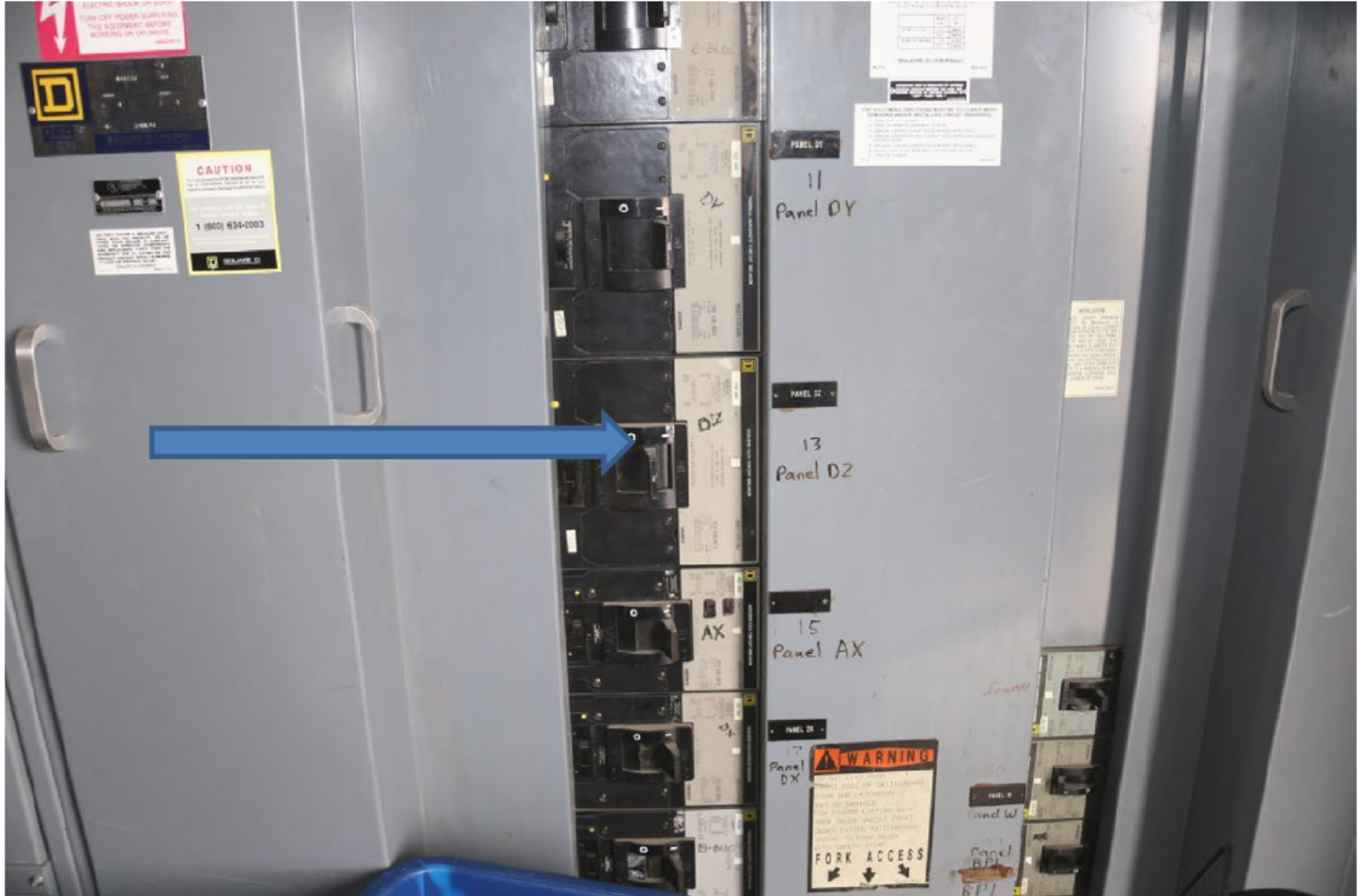
Blue arrow showing a trip on the main service panel. Picture is from file IMG_0313.CR2. A copy of this image is included in the addenda/held in the case file.
